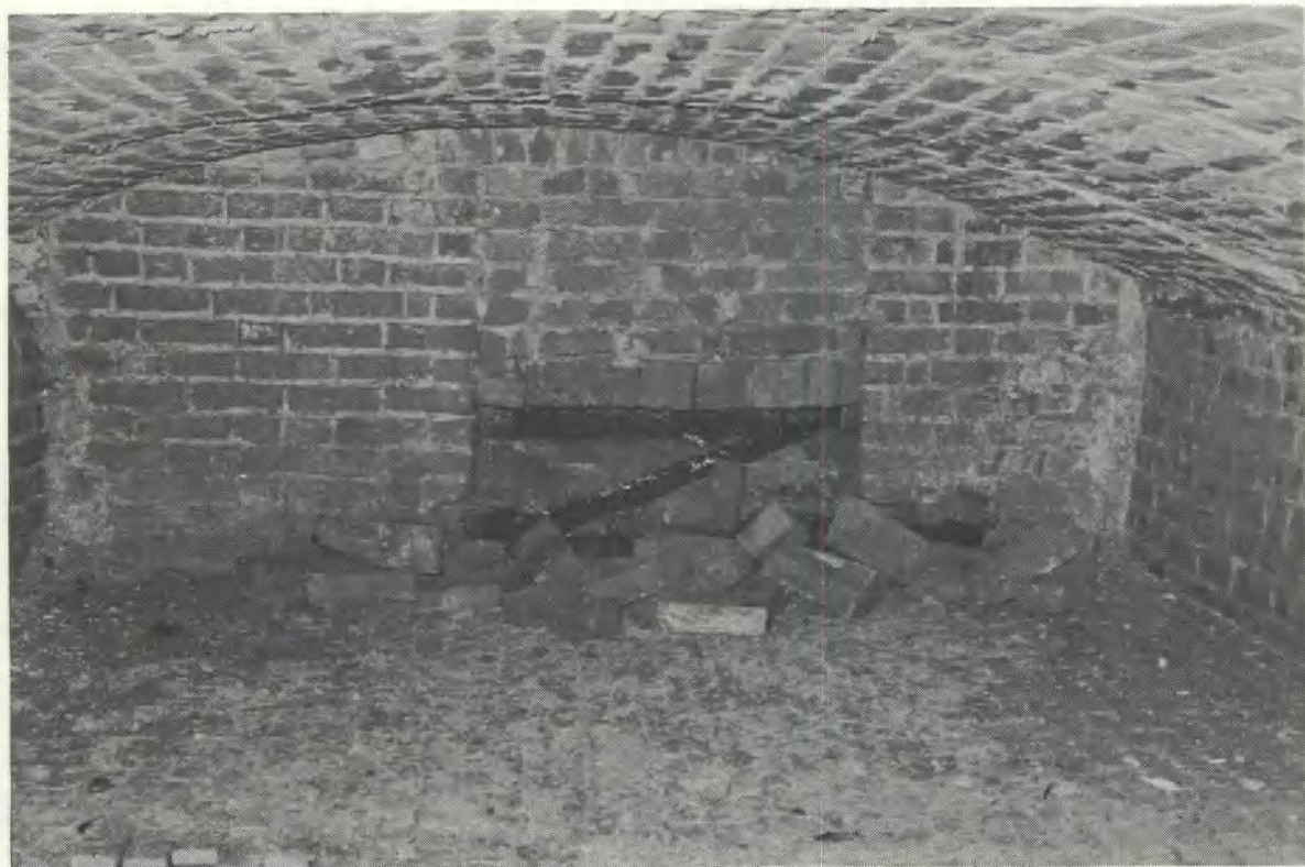
Plate 1 Brick Cistern at Stopsley
